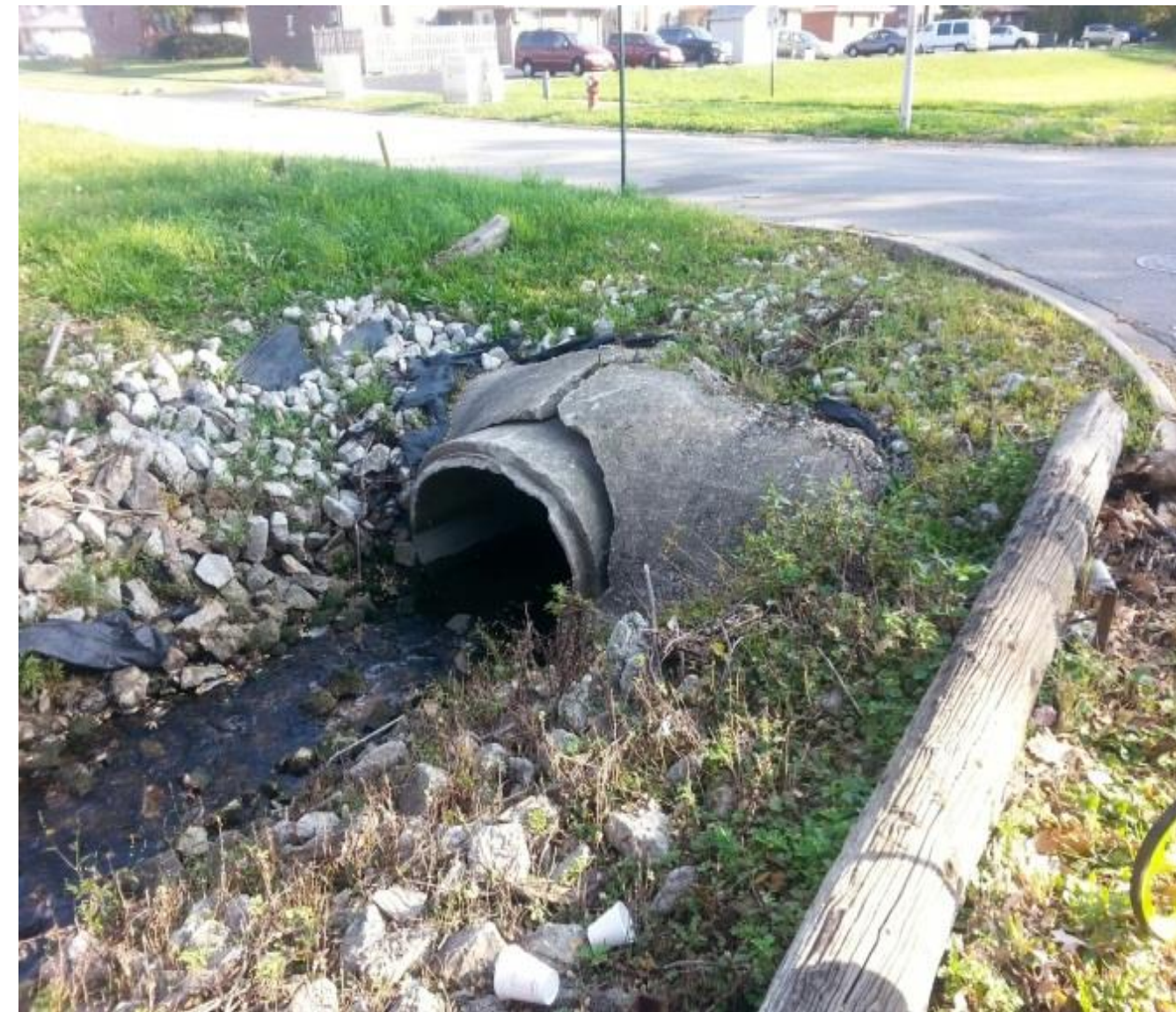
Left: Restrictive 149 th St. Culverts Right: Restrictive Kilpatrick Avenue Culvert at 149 th St.
