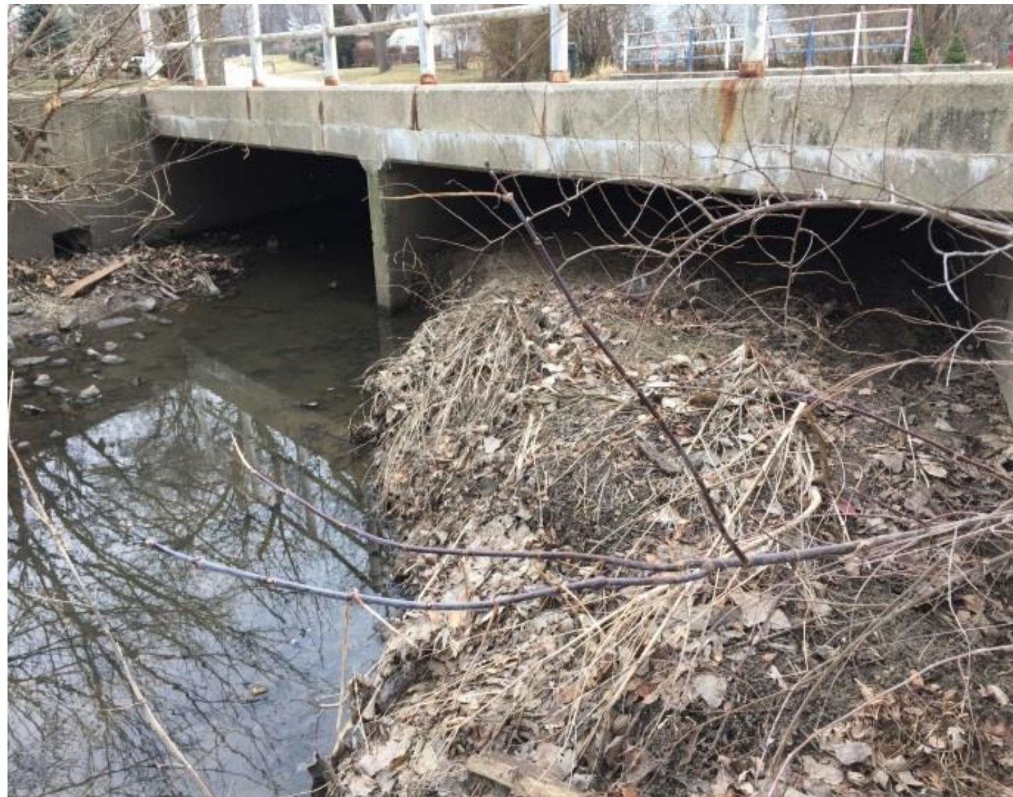
Left: Sediment Build Up at Laporte Avenue Right: Non-Engineered Rip Rap at Lavergne Avenue
