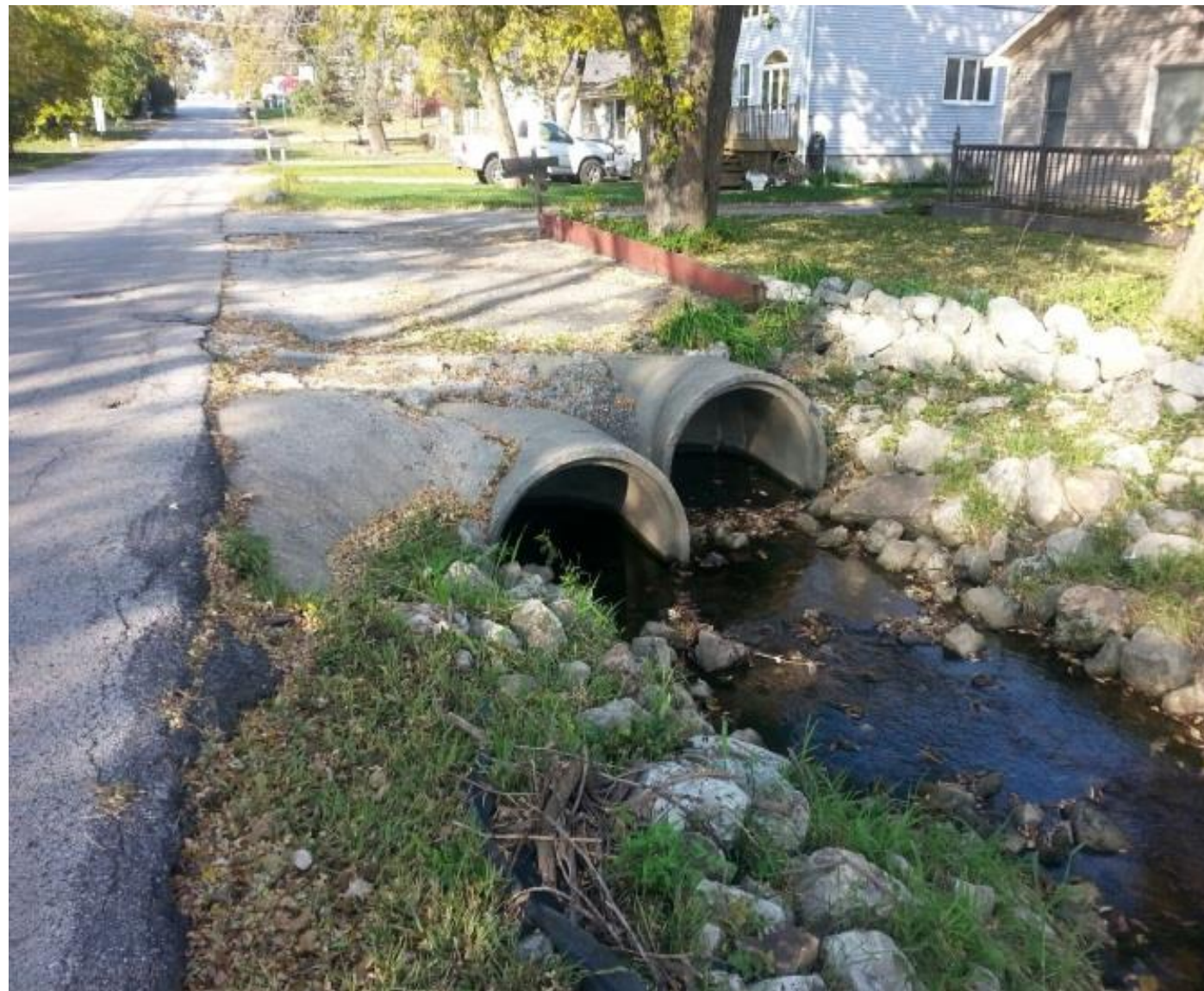
Left: Restrictive 149 th St. Culverts Right: Restrictive Kilpatrick Avenue Culvert at 149 th St.
