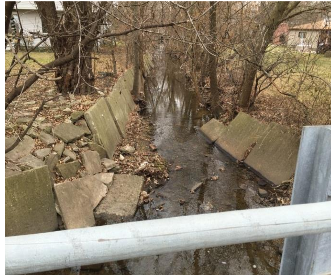
Left: Sediment Build Up at Laporte Avenue Right: Non-Engineered Rip Rap at Lavergne Avenue
